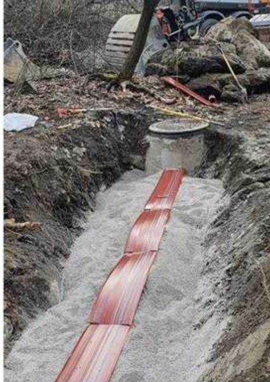
Figur 9d: Kabelmarkering.
